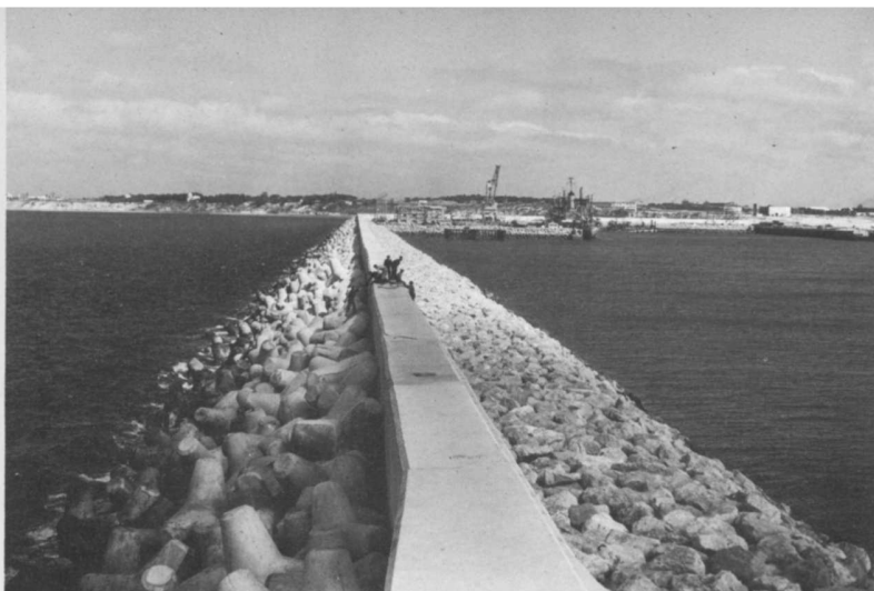
Tetrapods in place at breakwater in Rota, Spain
